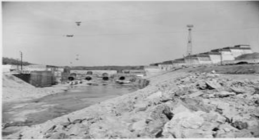
View, looking upstream, showing penstock monoliths and excavated tailrace.
